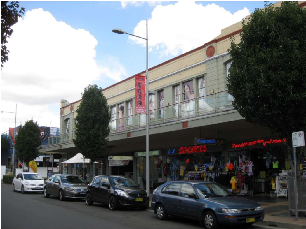
Figure 3: The site frontage of 197 Church Street.
