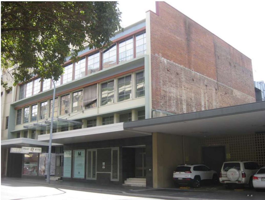
Figure 5: the view of 89 Marsden Street.
